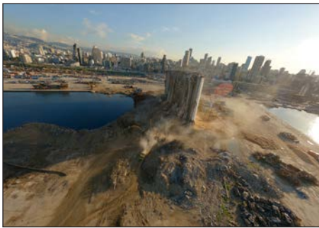
Beirut Blast: The Story of Warehouse 12
